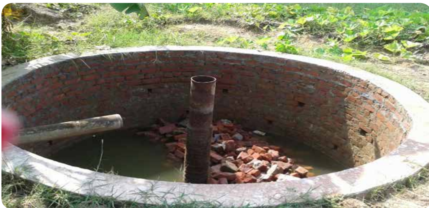
Rainwater harvesting Structures under Construction near Hostel 9
