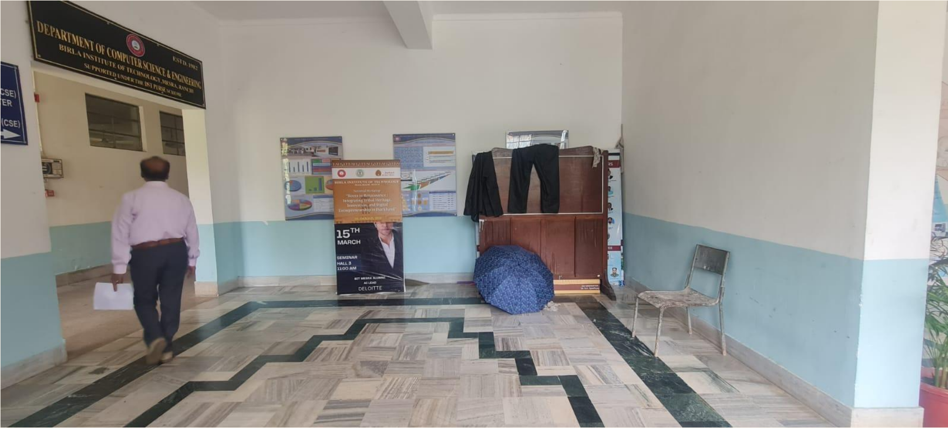
Existing : Left Side Smaller LOBBY
