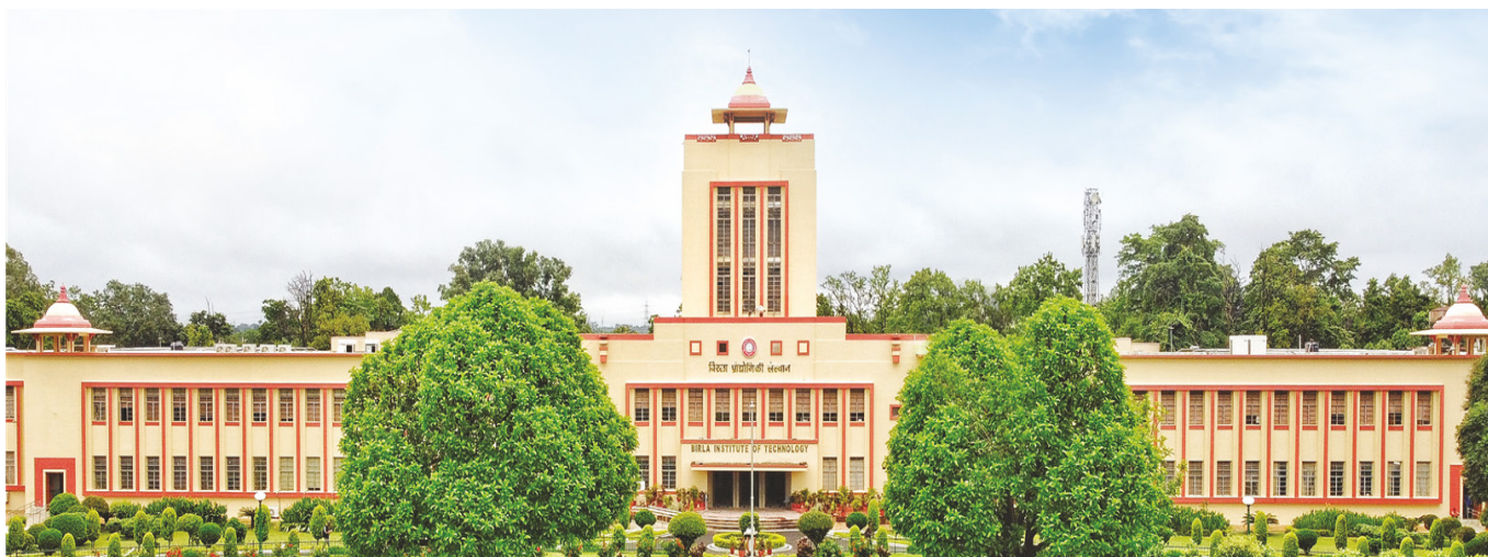
The Main Building at BIT, Mesra, Ranchi
