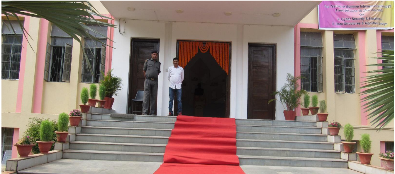
R & D BUILDING DEPARTMENT OF COMPUTER SCIENCE AND ENGINEERING
